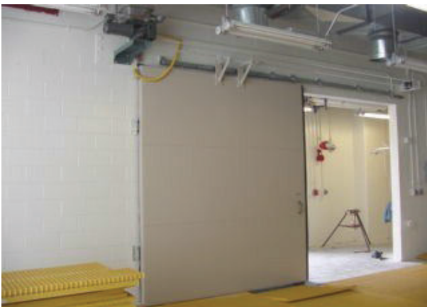
Blast and Fire Rated Sliding Door with Explosion Proof Operator for Chemical Storage
