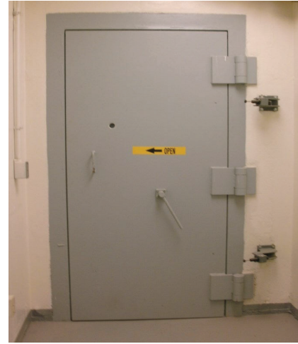
270 PSI Blast Door With Air Tight Seals and Sight Hole
