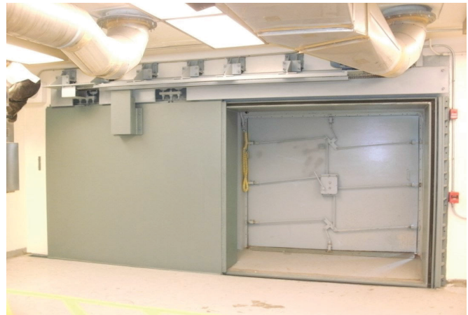
344 PSI Sliding Blast Door - Fragmentation Pneumatically Sealed- 15PSI Gas Tight Under Full Load Assumed to Act Simultaneously With the Shock Load.
