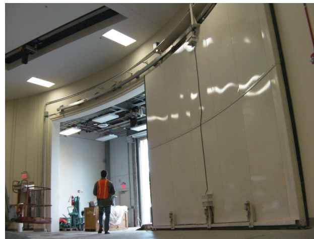
Curved Pressure Resistant Door STC 50 Acoustical rating
