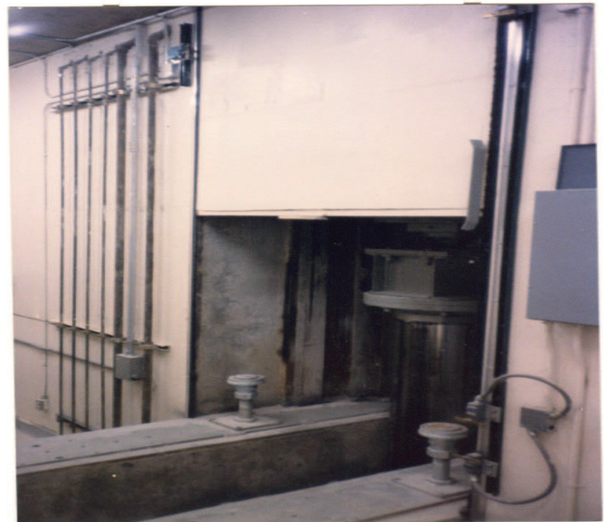
30 Ton Concrete Vertical Lifting Hydraulically Operated Door
