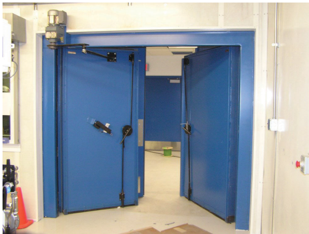
STC 60 Blast and Fragment Resistant Engine Test Cells Power Operators and Latches
